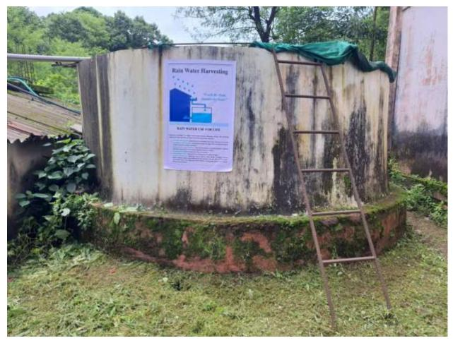
The college has an established rainwater harvesting system that captures and stores rainwater for reuse. This collected rainwater is utilized in the washrooms and toilets within the college premises. By integrating rainwater harvesting, the college reduces its reliance on external water sources and promotes sustainable water management practices. This system helps conserve water, reduces utility costs, and supports the college's commitment to environmental sustainability.
