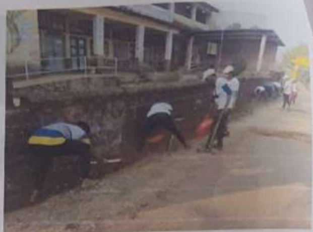
112-feet-long sewer along the road was cleared
